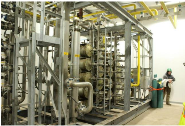
Methane from dairy manure runs through a system of membranes at the DTE Vantage biogas facility. It cleans it of oil, water and unwanted gases before sending the natural gas to a transmission pipeline 8 miles away. Tri-State Neighbor photo by Janelle Atjeo
