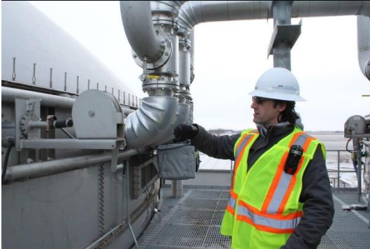
Dave Grooms, plant technician at the DTE Vantage biogas facility near Beresford, S.D., explains the process to breakdown dairy manure in a 2-million-gallon anaerobic digester. Tri-State Neighbor photo by Janelle Atyeo
